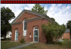
South Glastonbury Library on High Street
